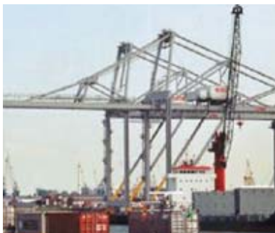
Ship-to-Shore cranes Rotterdam
