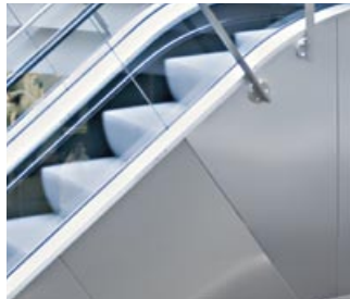
Stainless steel cladding
