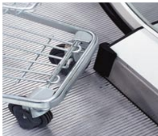
Trolley protection in autowalks
