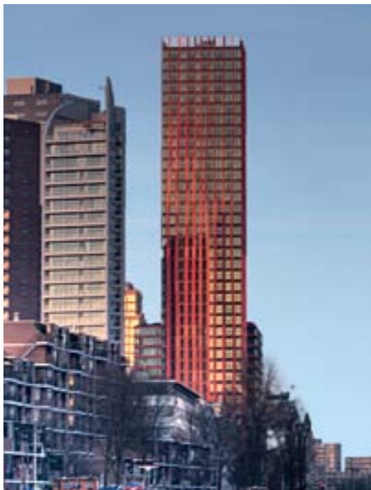
Red Apple, Rotterdam, the Netherlands High-rise residential building with 2 KONE JumpLifts.
