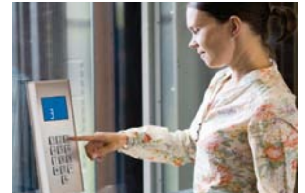
The Destination Operating Panel can work as a directory showing the different wards. When the user enters the lobby, he or she selects the destination on the Destination Operating Panel. The DOP indicates which elevator will be available. When the elevator arrives, it automatically takes the visitor to the desired floor.
