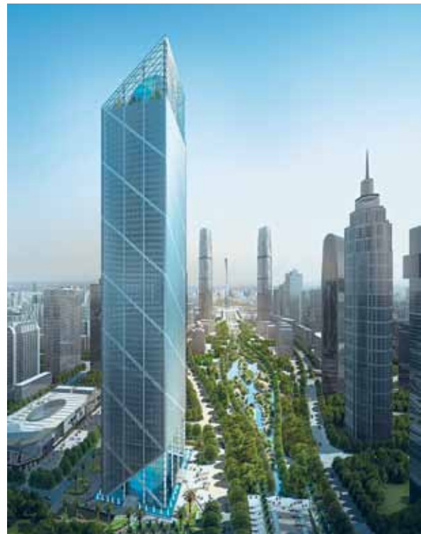
KONE is involved in green building projects around the world. The 303-metre-high Leatop Plaza building in the Chinese megacity of Guangzhou is a shining example.
