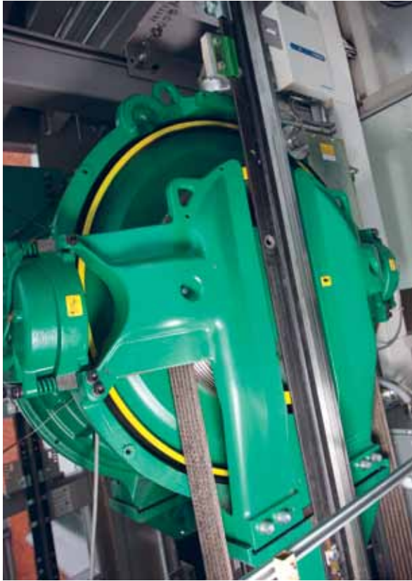
The energy-efficient KONE EcoDisc hoisting machine.
