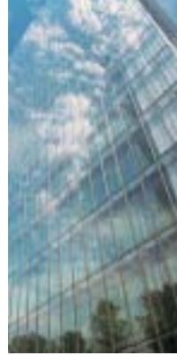
KONE Head Office, Espoo Designed by Anti-Matti Siikala. Features four KONE Alta Scenic elevators at a speed of 2.5 m/s.
