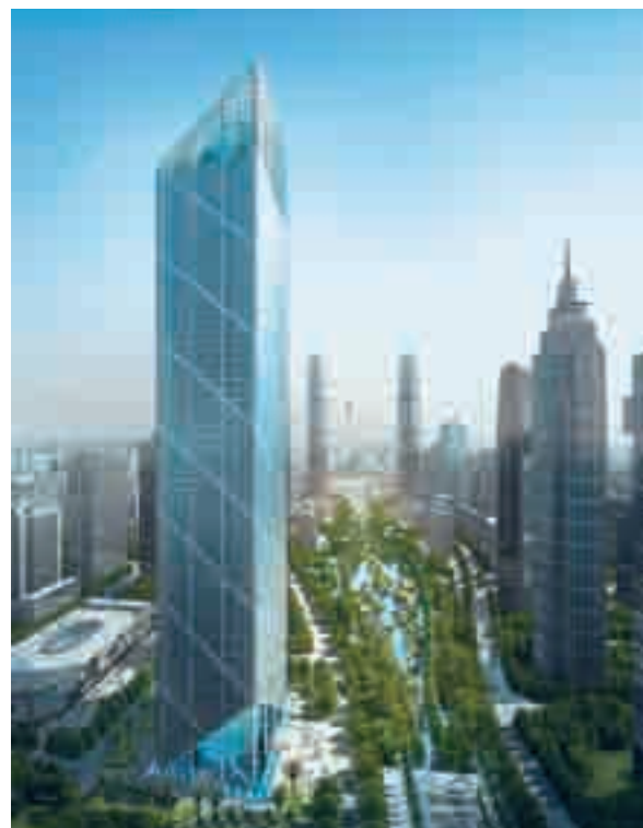
KONE is involved in green building projects around the world. The 303-meter-high Leatop Plaza building in the Chinese megacity of Guangzhou is a shining example.
