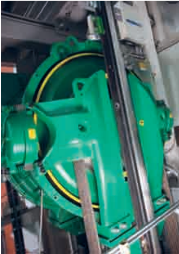
The energy-efficient KONE EcoDisc hoisting machine.
