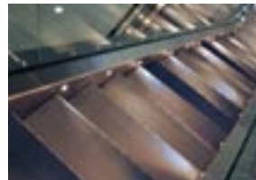
LED skirt lighting
