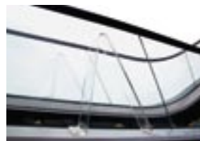
Anti climb barrier
