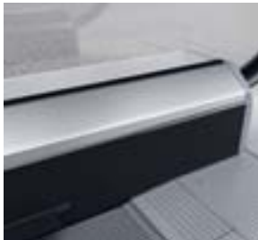
Sheet steel skirt with black anti-friction coating
