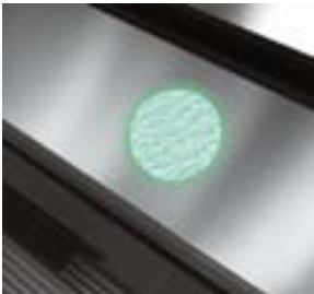
Traffic lights located in the decking
