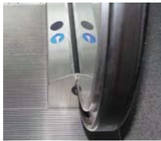
Traffic lights on decking
