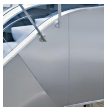
Stainless steel deckings and cladding
