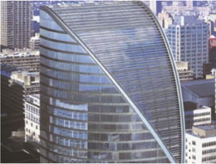
Moorhouse, London, UK
