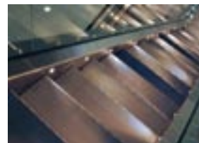
LED skirt lighting
