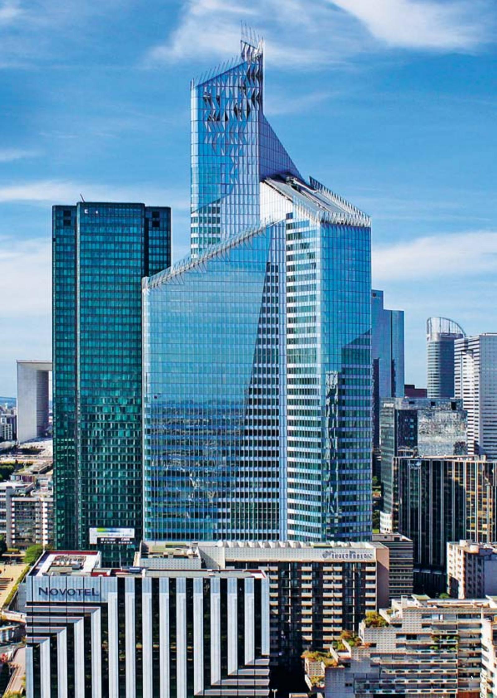
Their plan was ambitious. The changes needed to be dramatic, but done quickly in a congested area of Paris. Rather than demolish the existing tower, the building would be stripped down and a new tower designed and constructed around the old metal framework. All this was achieved in remarkable time – just four years, from 2007 to 2011.
