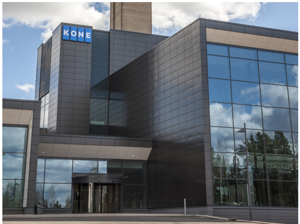
KONE's People Flow Center in Hyvinkää, Finland, is LEED Gold certified.
