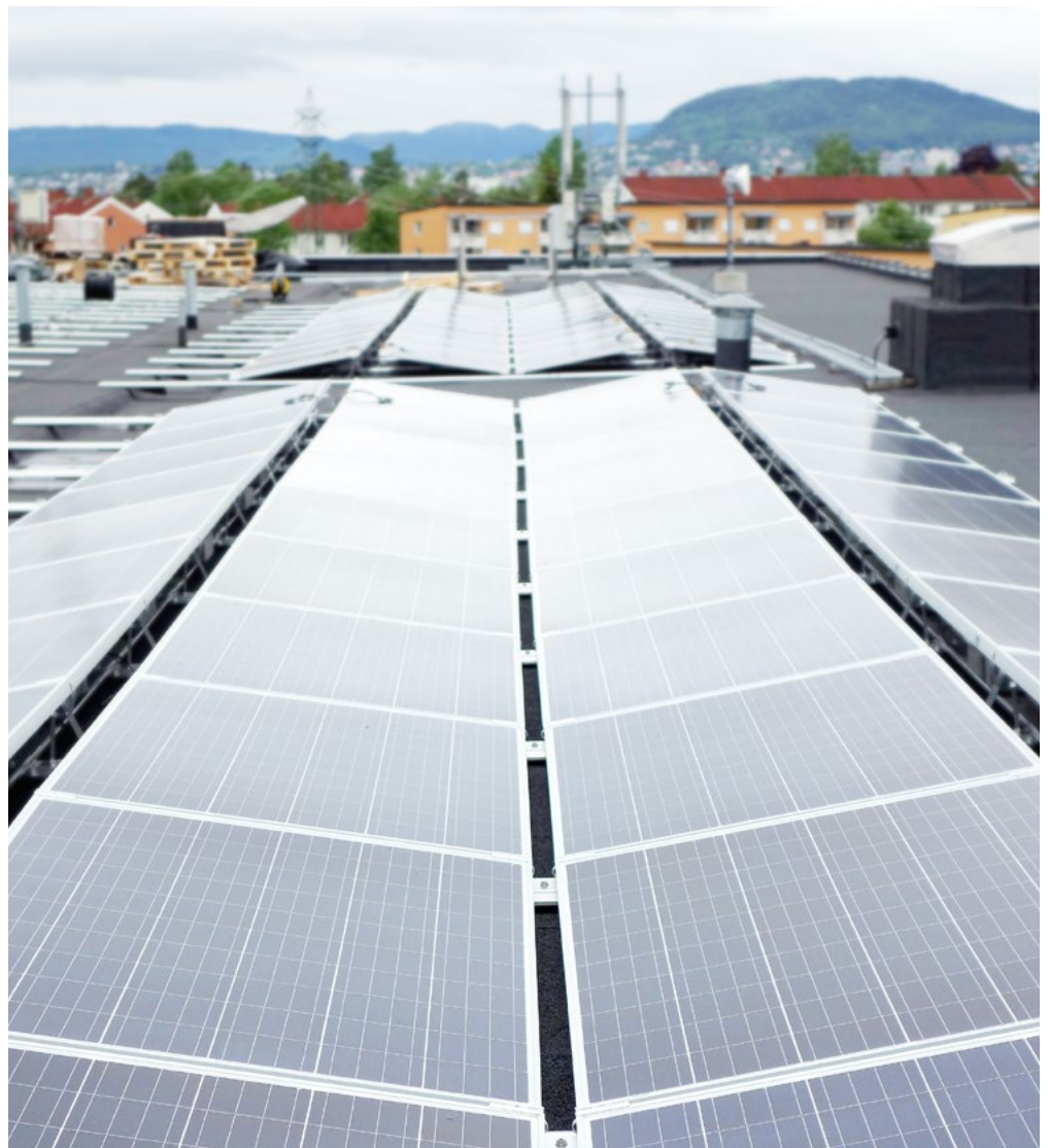
In May 2016, 180 solar panels were installed in KONE Oslo's passive energy house covering one third of the rooftop.
