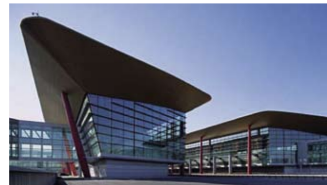
Capital International Airport Extension, Beijing, China
