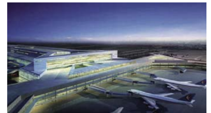
Hongqiao airport Extension and Transportation Junction Project, Shanghai, China
