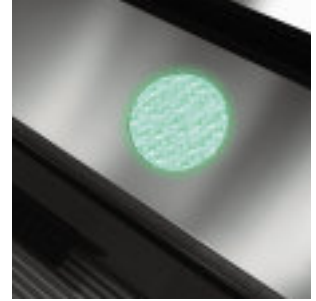
Traffic lights located in the decking
