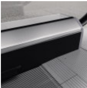
Sheet steel skirt with black anti-friction coating
