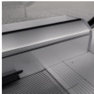
Brushed satin stainless steel skirt with clear anti-friction coating
