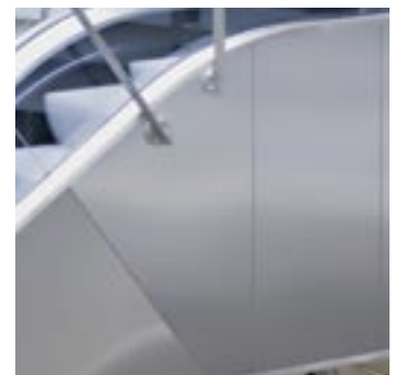
Stainless steel deckings and cladding
