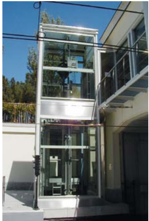
Figure 3. Self-standing steel shaft
